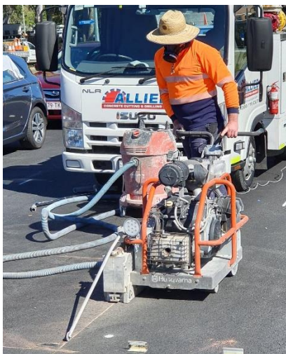
Figure A.5: Loop cutting road saw (Husqvarna FS 400 LV)
